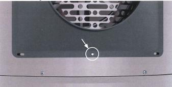
Secure the left side of the duct adapter with two (2) of the remaining screws starting from the top utilizing the duct adapter holes along its perimeter.
