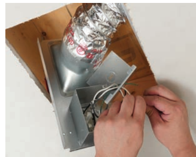
Wiring and Duct Installation Made E-Z
